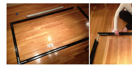
Check alignment, then tighten screws. Confirming with your fingers that the joints are aligned nicely, go ahead and tighten the remaining set screws.
