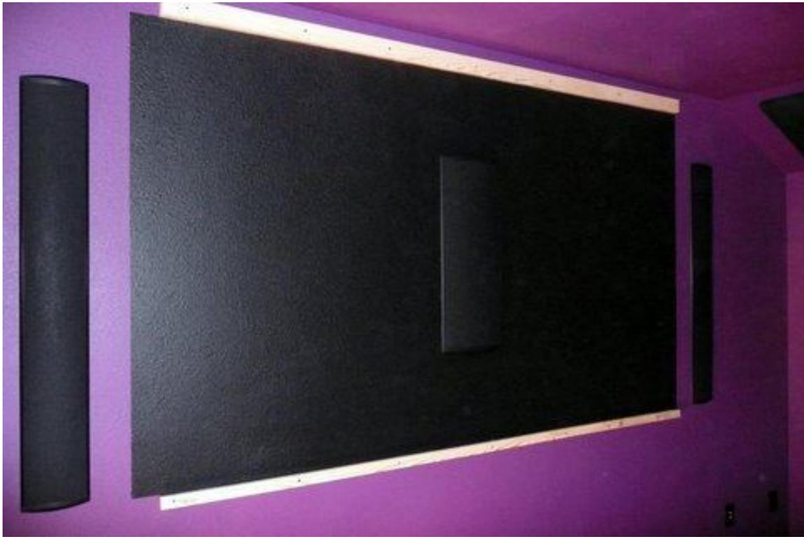
I highly recommend painting the area behind the screen a flat black to keep light from reflecting off the wall and bouncing back through your screen material degrading the picture.
