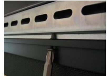
5) Locate the bag in the white remote box that has the five stainless steel truss head screws. Grab a level and mount the DIN rail to your wall using these screws. If you have a very curvy wall, you can space out a screw or two with washers or shims. You don't want the DIN rail to be curvy, or else the case won't engage all the way. Make sure at least three screws are securely mounted into a stud.
